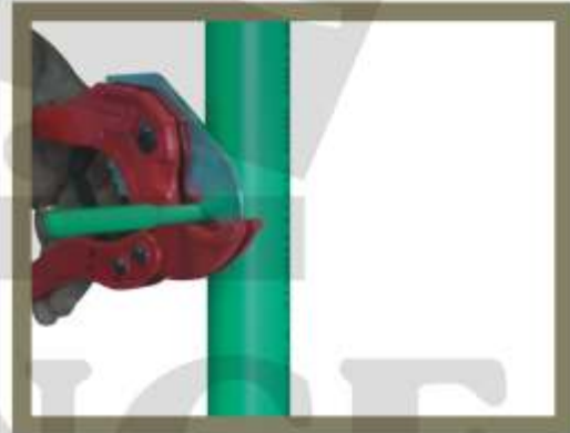
After cooling, cut the repair bar projected outside the pipe line using pipe cutter. Kindly do the needful in case the printing is not yet started.
