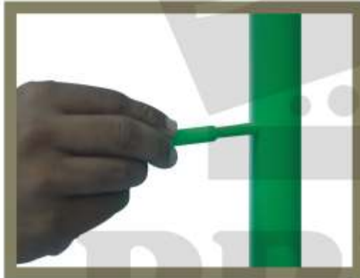
Insert heated repair bar in the hole up till the full depth and hold it for a minute.
